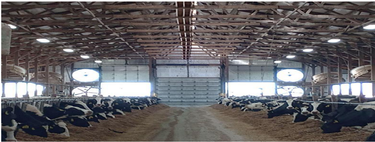
Photo 23: (Source: Photo by University of Wisconsin–Madison). Tunnel-ventilated dairy buildings.
