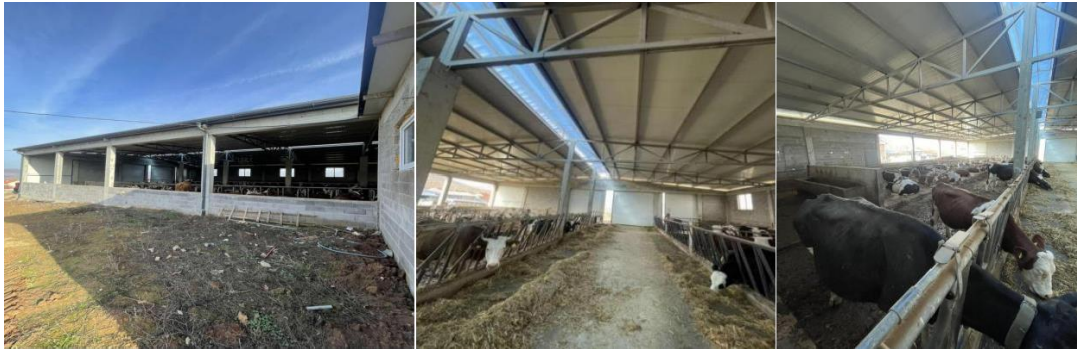
Photos 11, 12, 13: (Photo: Muhamet Shala, 2025, Kosovo). Farm with sidewall openings and natural ventilation (dimensions: 29 m L ×
